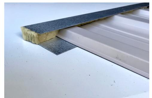
Cut wall sheet approximately 10mm shorter than the top of the roof sheet profile, then install the Barge B.A.L Flashing over cut ends of wall sheet and push down to be level with the top of the roof sheet profiles, compressing the rockwool insert. Can cater for approximately 20mm of variances.
